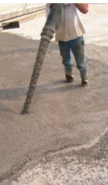
Pumpable Argex concrete (HST- Merksem)
