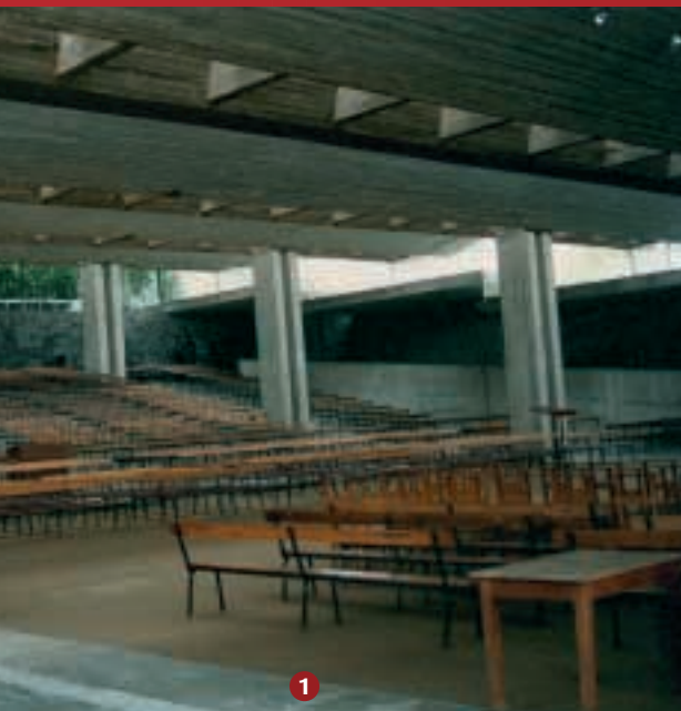
Ceiling construction in light structural concrete (Place of pilgrimage - Beauraing)
