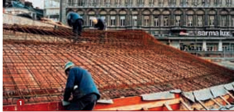
Archeoforum in structural lightweight concrete (Place St-Lambert - Liège)
