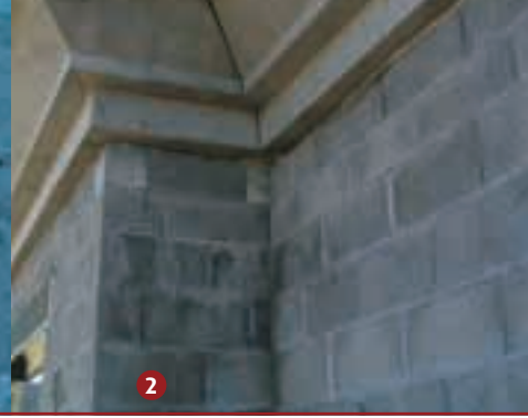
Prefab cornices in lightweight concrete
